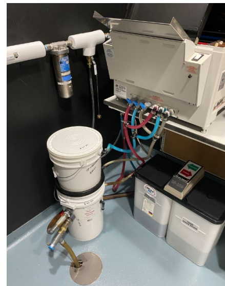
Figure 2: SIU inspection of silver recovery unit
